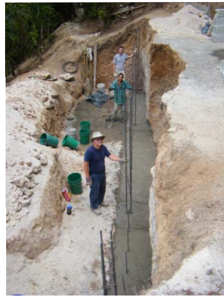
The completed footing for the lower level.
