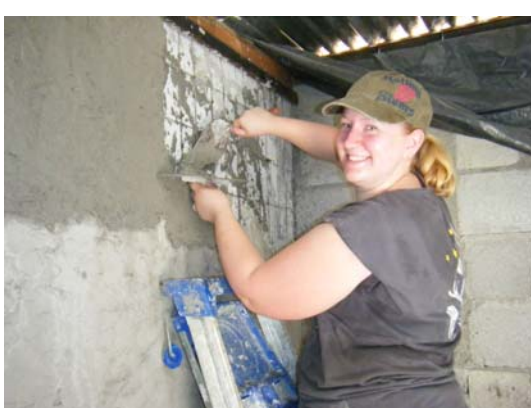
Stuccoing the Ministry Building
