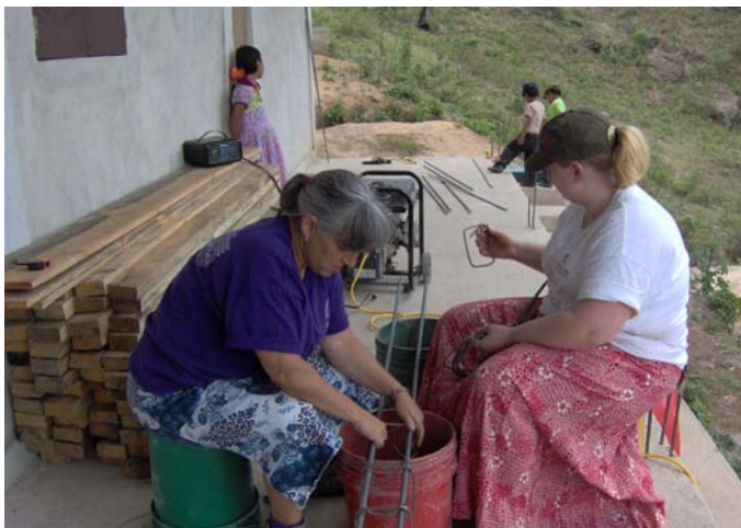
Robin and I trying the steel for the column forms.
